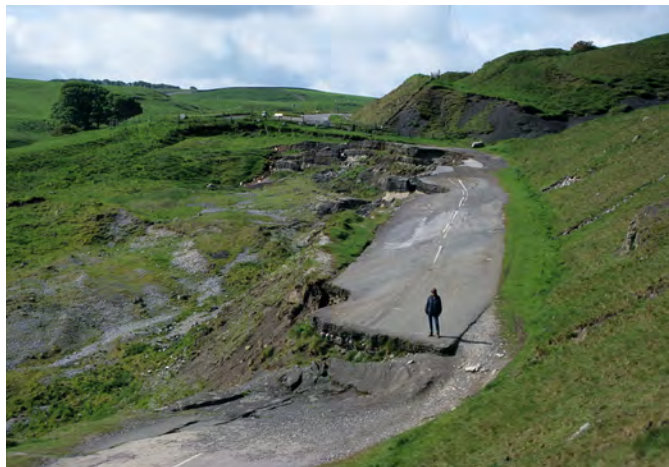
The road across the middle section of the Mam Tor landslide, where currently active displacements of the various fault slices are clearly shown by offsets of the road surface, which has not been maintained since its closure in 1979. (Photo: T. Waltham).
