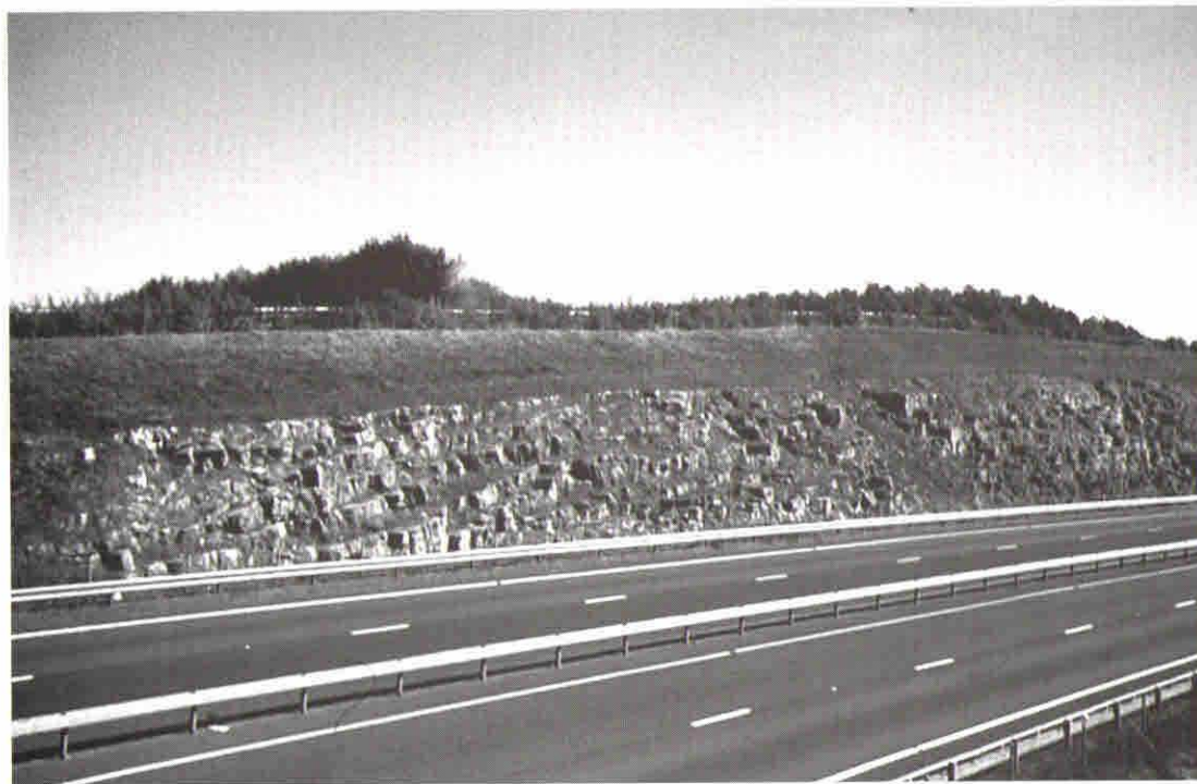
Figure 2. Photograph of section NE taken from section SE showing how fault fractures within the White Limestone Formation have produced dip and fault blocks with varying dips, all contra to the regional dip. The latter is at a very low angle from left to right.
